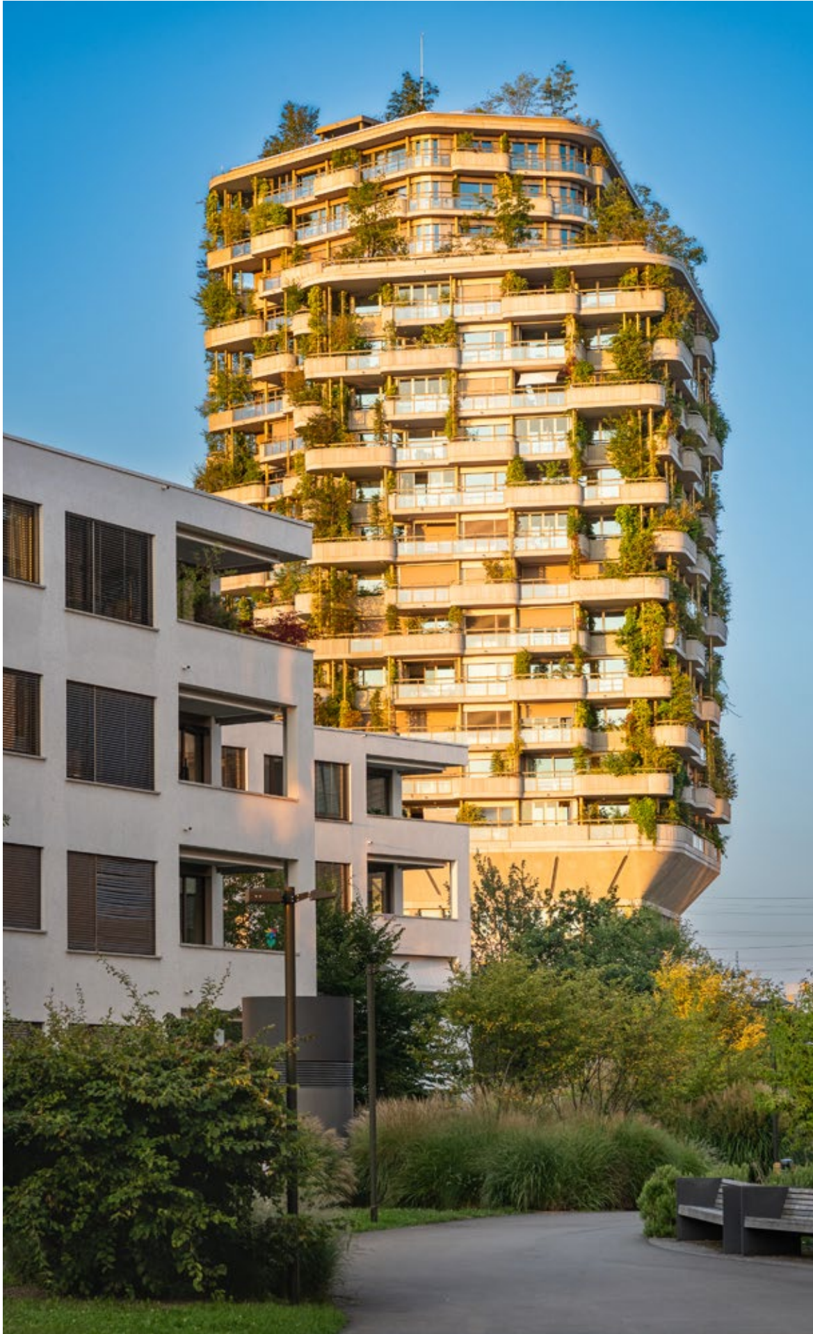
Aglaya garden high-rise, Suurstoffi site, Risch-Rotkreuz
